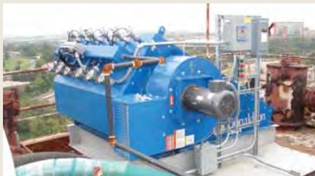
CPV Multiple cement silos 4,800 cfm
