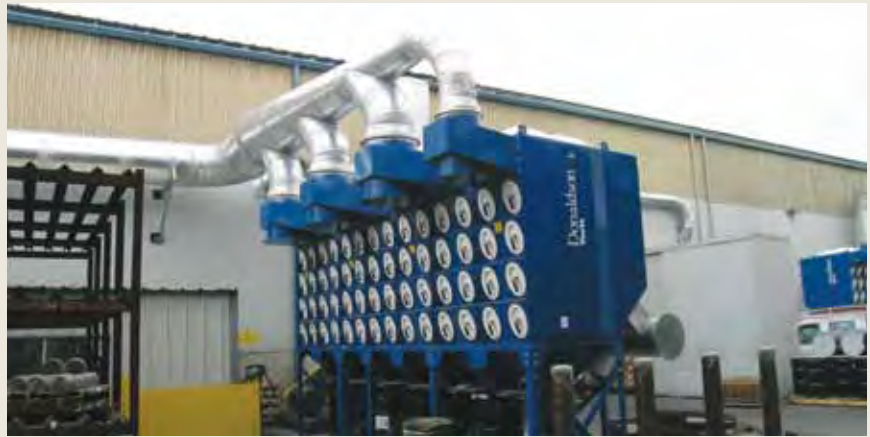
DFO Grinding 74,000 cfm
