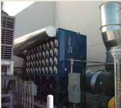
DFO Welding fumes 53,000 cfm Left: outside Right: inside
