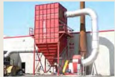
MB Glass processing 25,000 cfm
